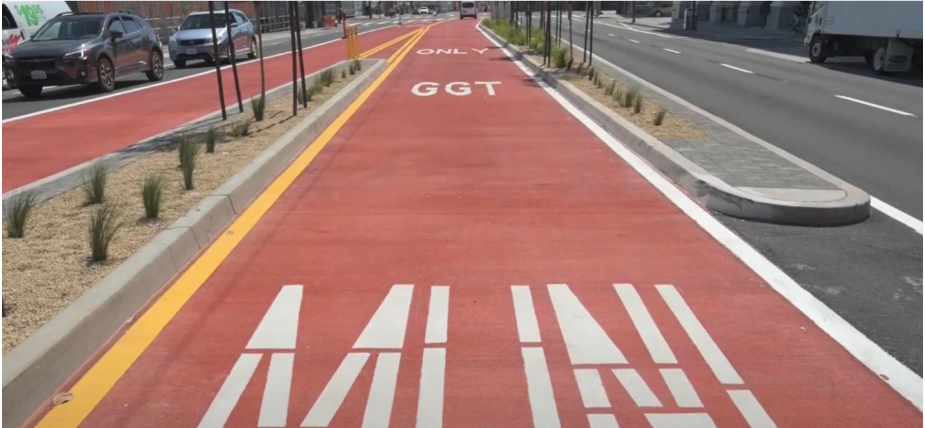
Transit lane separation for Muni on Van Ness Avenue in San Francisco (source: SFMTA).
