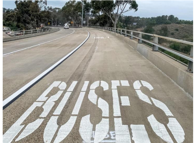
Part-time transit-only lane on SR 94 in San Diego (source: CSET).
