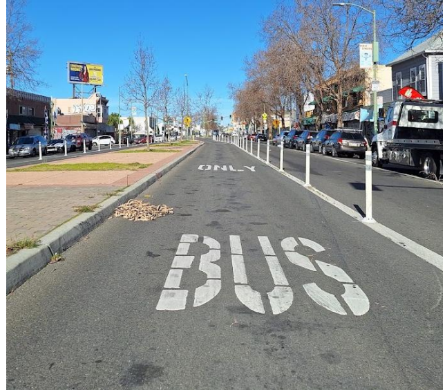
Transit lane separation on SR 185 in Oakland (source: Caltrans).
