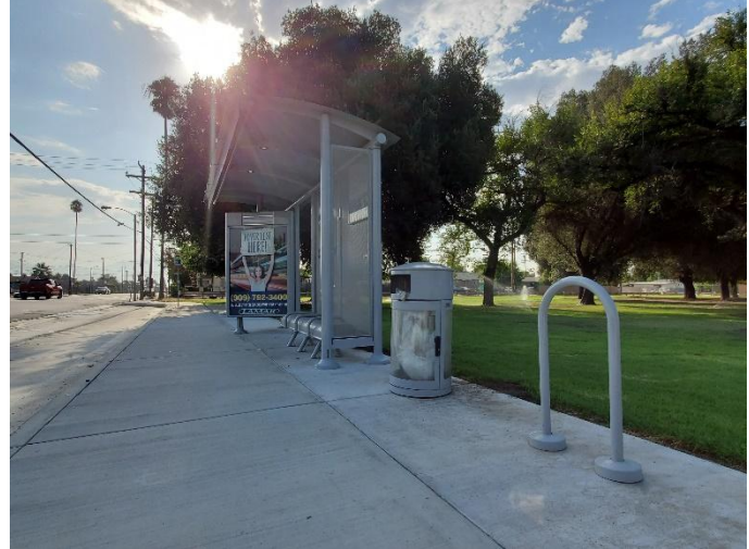
Bus stop accessibility improvements on SR 66 in San Bernardino (source: CSET).
