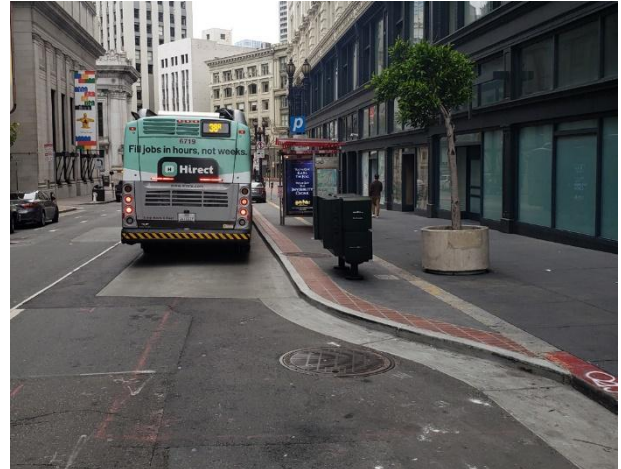
Bus bulb on O'Farrell Street in San Francisco (source: SFMTA).
