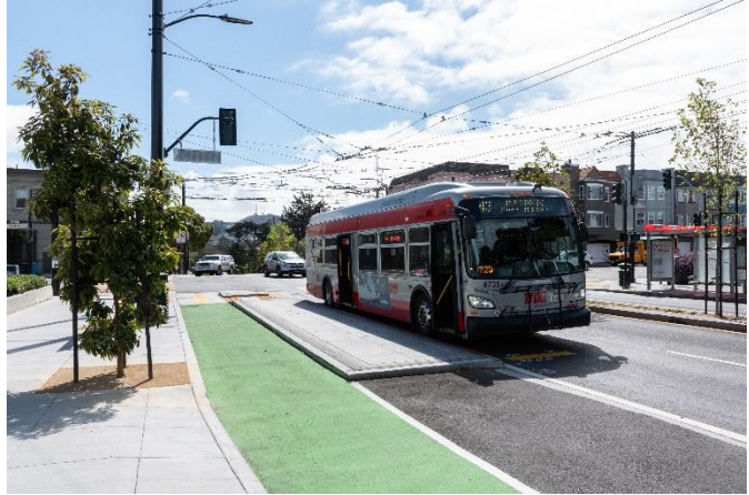
Bus boarding island on Masonic Avenue in San Francisco (source: SFMTA).
